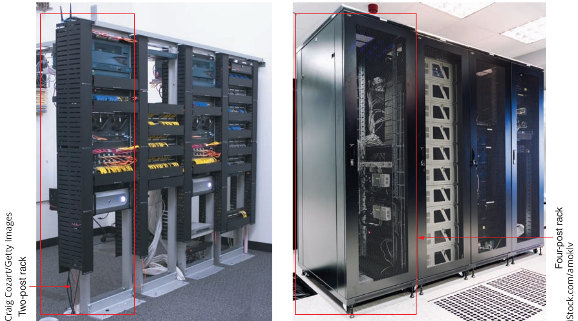
Figure 2-11 Open two-post racks and enclosed four-post racks
