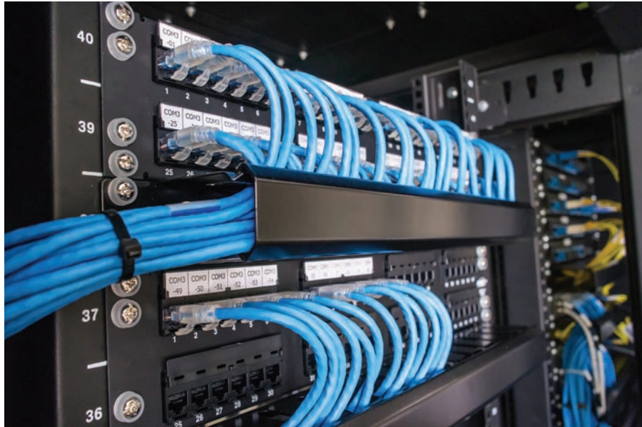
Figure 2-5 Patch panel on rack
