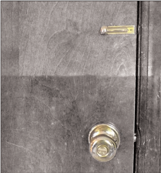
FIGURE 7.7 A “helper” has been added to the lock on the door knob to increase security.
