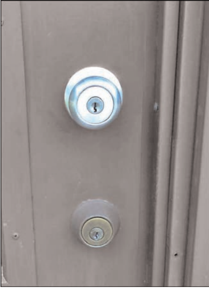
FIGURE 7.8 Adding two actual locks to the door effectively increases security.
